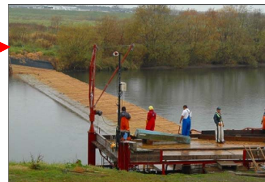
The weir at Tokoro Estuary traverses the river completely. This style is common in Hokkaido.
